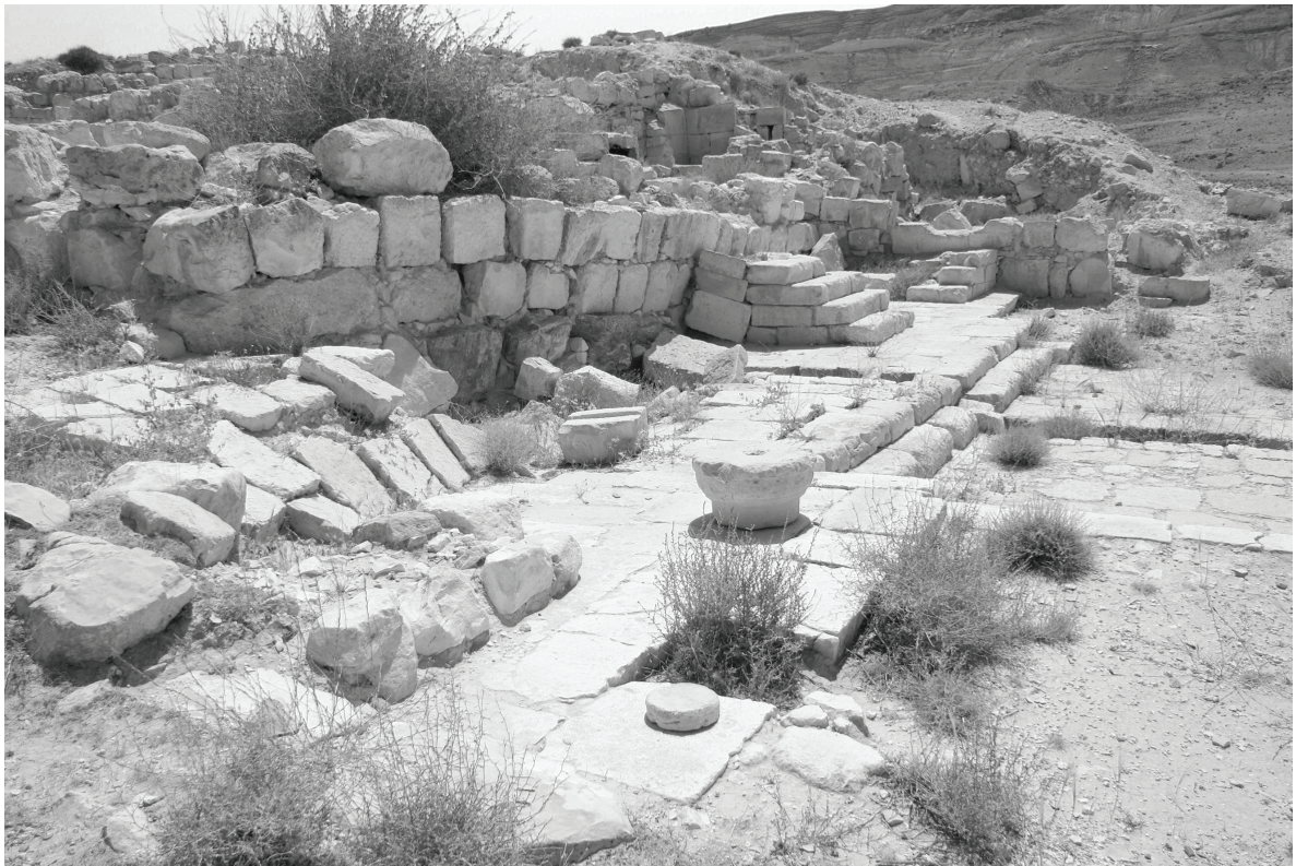
Fig. 6. Façade of room (J) and the upper part of the esplanade (S) deformed by and earthquake (photo P. P.-F. 2007)
